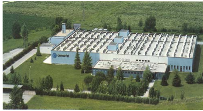
COMEFRI SpA factory at Artegna (UD) – Italy with 6.300 m 2 workshop. Production of industrial fans and special executions. Test facilities: laboratory accredited by AMCA.
